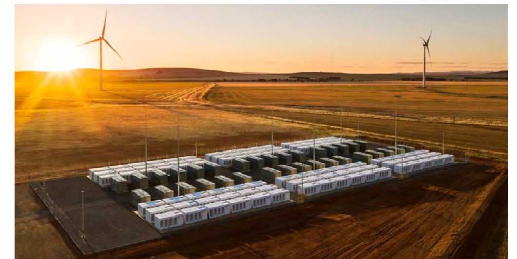
The battery at the Hornsdale Power Reserve, South Australia.
