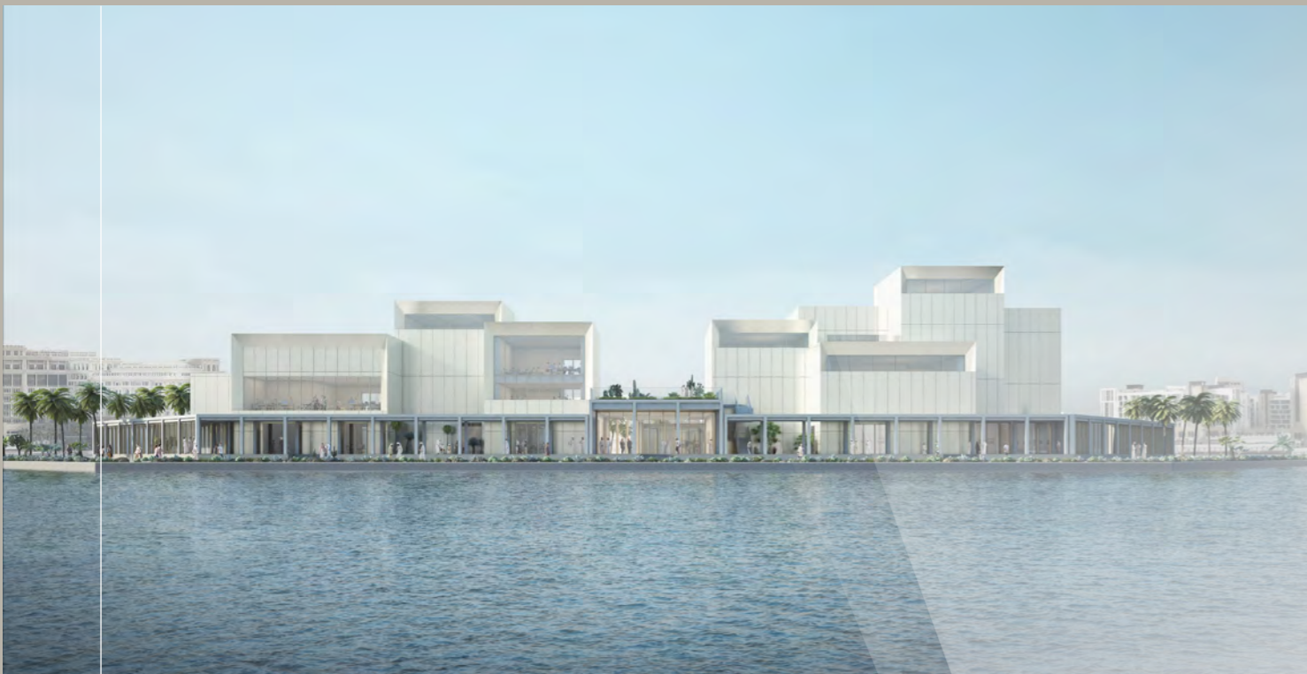
Jameel Arts Centre - Dubai, Northside View, from the Creek, © Serie Architects
