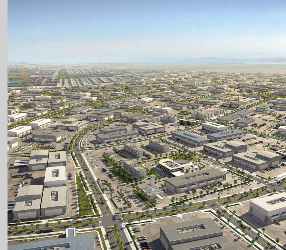
Right: KAEC Industrial Valley in Saudi Arabia
