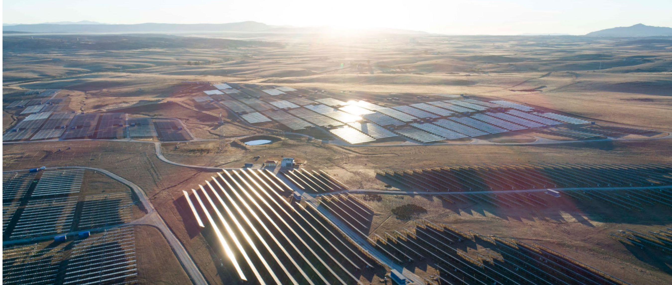
The 46.20 ha FRV constructed solar farm in Trujillo (Extremadura) Spain, (now owned/operated by Vela Energy) with 11.55 MWp capacity and an annual production of 21,959 MWh/pa supplying 6,297 households and avoiding 7,153 tonnes of CO 2 annually.
